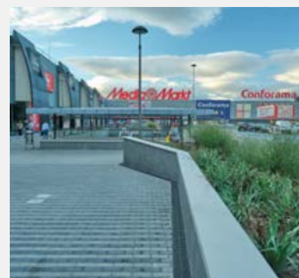
Rivas Futura: pavements and pedestrian access.
